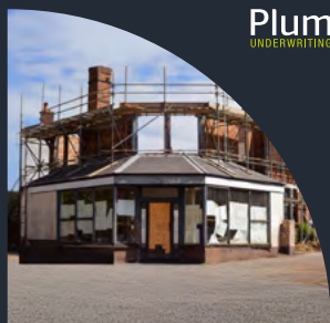
Commercial Building Works
